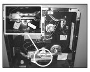
Water heater drain plug location
